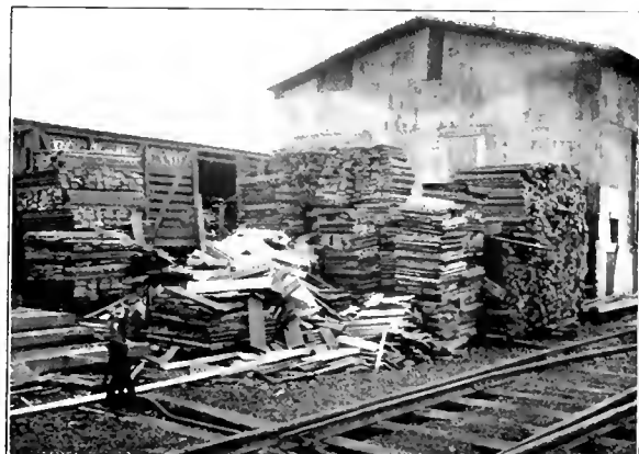
Reclaimed Roofing, Siding and Decking Ready for Use
